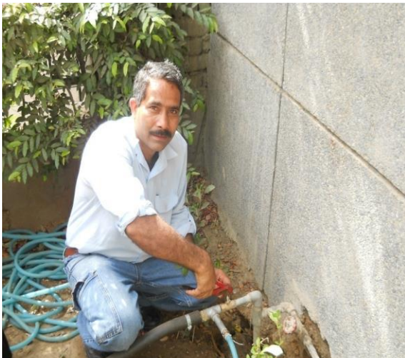
Approximately 10 house with plumbing leakages in the complex were rectified by the plumbers of the hotel.
