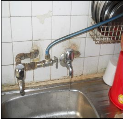
A leaking tap in the kitchen of one flat...
